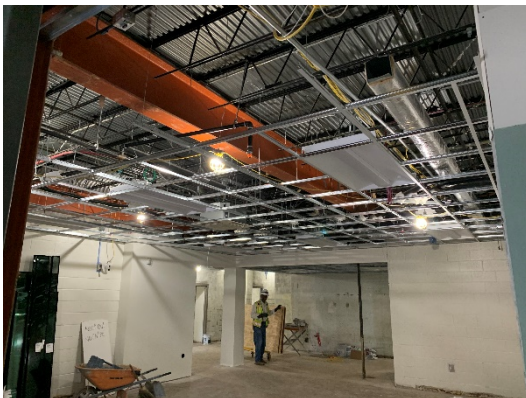
Ceiling Grid and Lights in building 2040
